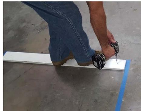
After the first sill plate is anchored to the floor, anchor the second measuring off of the first to ensure that they are set square. This is very important; if the sill plates are not square adjust them to make them square.
